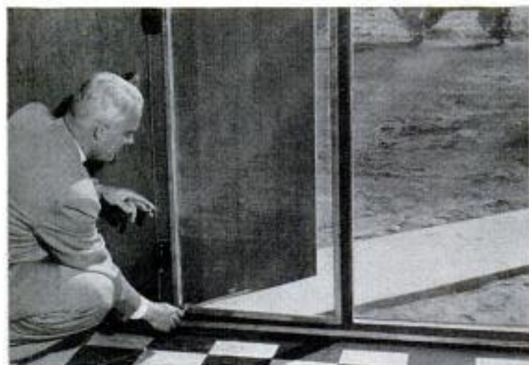
Cox operates a window opener that has been attached to panel in small unit built to serve as guest house or motel unit. Glass window panel at right is part of wall, does not open
